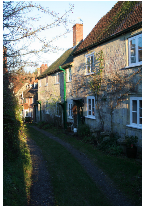
4. Looking East through Bakehouse Yard
