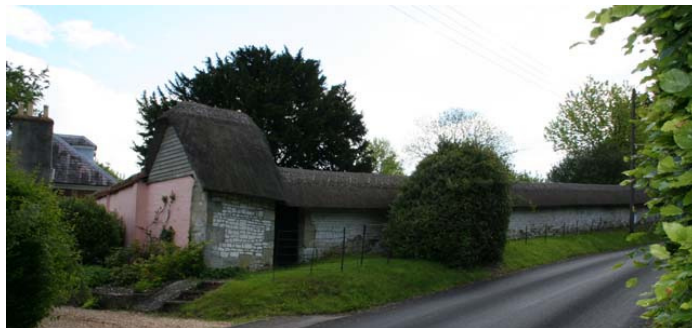
Thatched "block chalk" wall on Stops Hill
