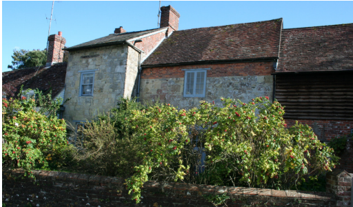
Mill House, The Dene
